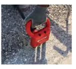
Concrete scabbling using single-head, Vibro-Lo™ Scabbling Hammer
